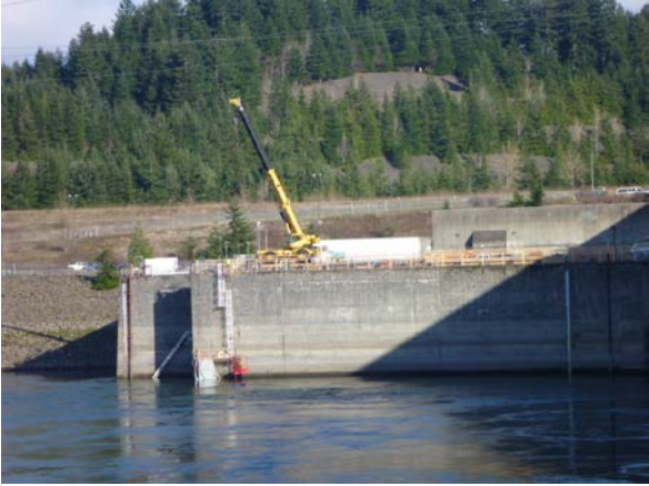
WA Shore LPS Construction.
