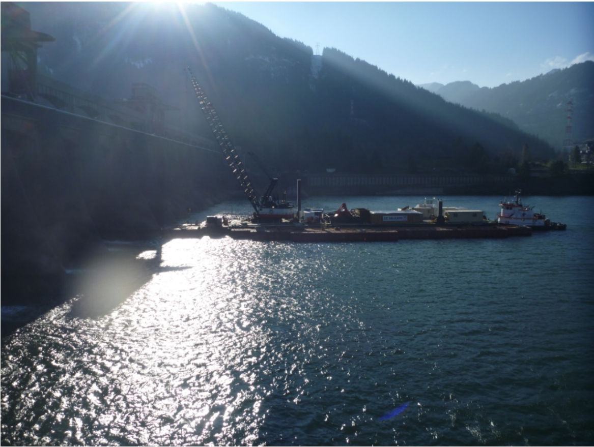
Spillway Erosion Repair.
