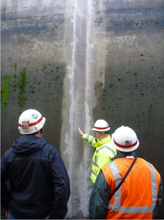
B2CC Joint Repair.
